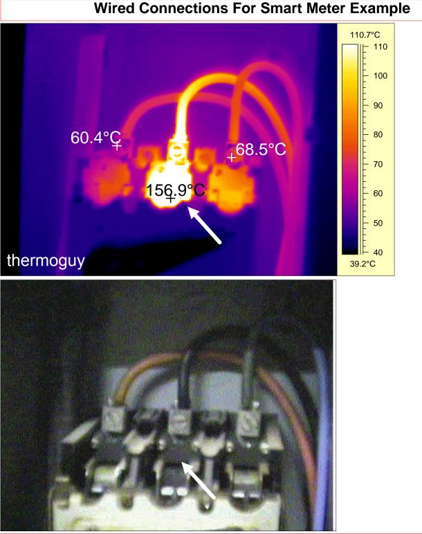
Electrical Meter Bases have wired connections as well as stabs. Qualified electrical professionals would check ALL connections when the meter is pulled.(safely and working with the home owner) Before installing the new meter any electrical problems would be identified and repaired, even replacing the meter based if required. There are no compromises electrically or there will be failure with consequences that include fires that may happen immediately or later.
