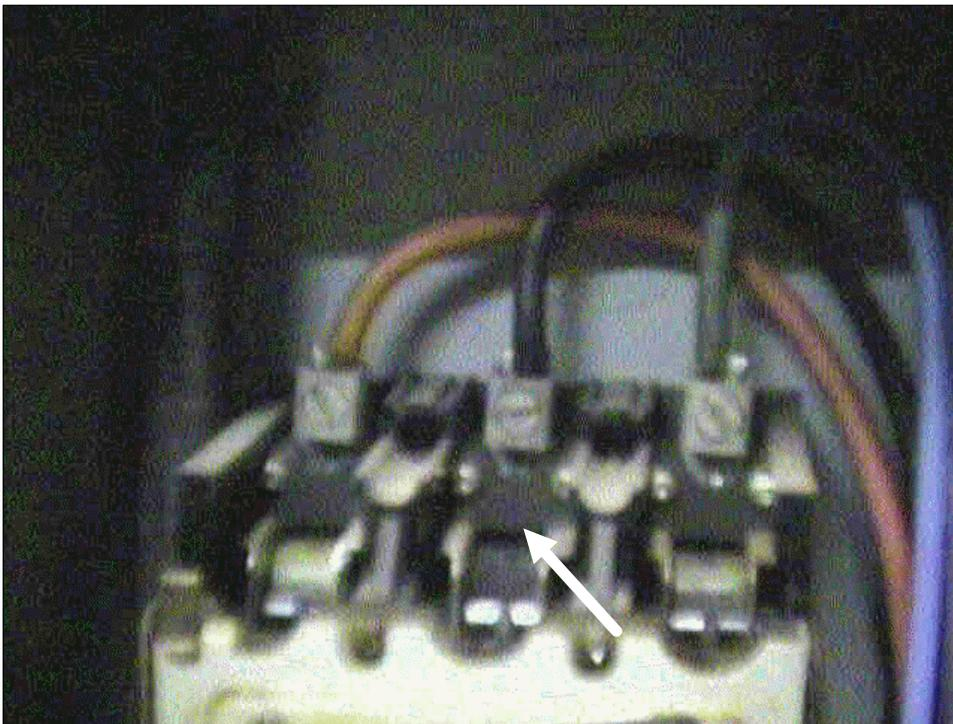
Electrical Meter Bases have wired connections as well as stabs. Qualified electrical professionals would check ALL connections when the meter is pulled. (safely and working with the home owner) Before installing the new meter any electrical problems would be identified and repaired, even replacing the meter based if required. There are no compromises electrically or there will be failure with consequences including fires.
